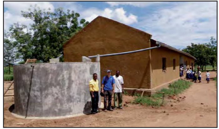
A rainwater tank almost finished by EI at Uhambingeto Primary School
