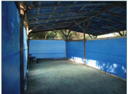
Temporary school structure
