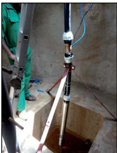
**The solar powered pump being installed in the pump sump**
