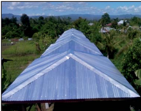
The roofs are on.
