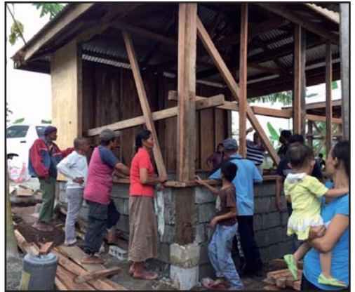
A house nearing completion.
