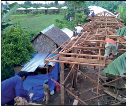
The wooden frames being erected.
