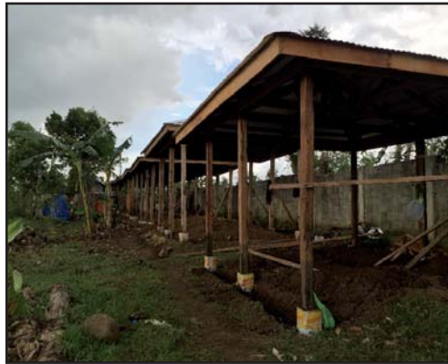
The wooden frames being erected.
