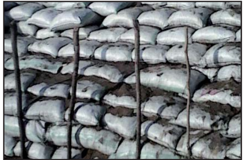
Water protection bund to slow down the flow of water in riverbeds and flood-prone areas
