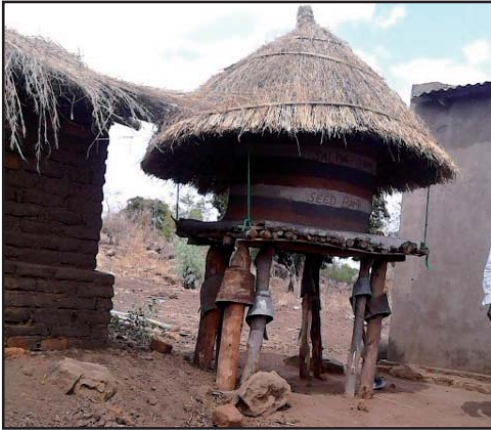
An ngokwe , a traditional maize storage facility with a new touch (metal around the legs to keep the rodents out).
