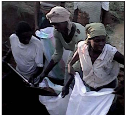
Ladies working on a bund construction
