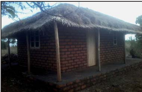
Rebuilding 184 homes destroyed in floods (to date 160 one room homes have been built)
