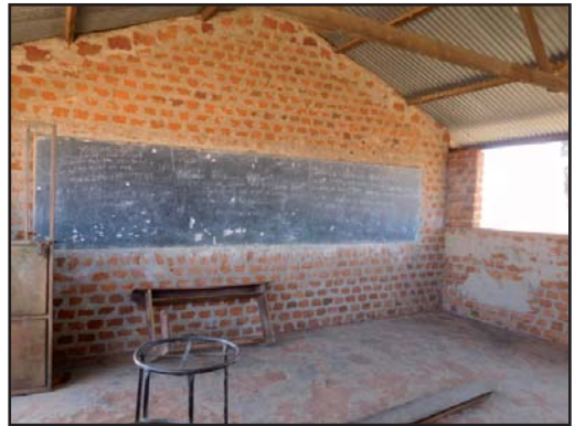
One of the classrooms
