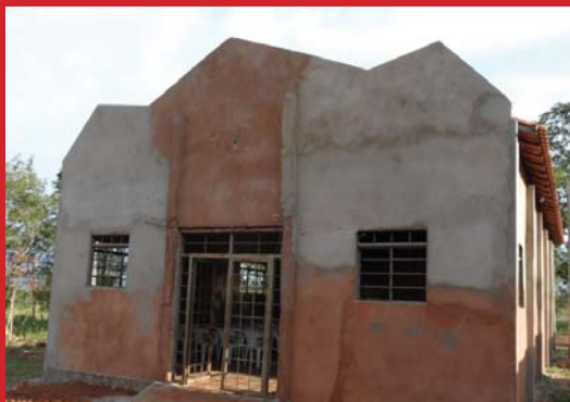
Progress on the church building
